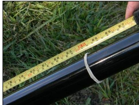
impaired if the Ground Post is leaning sideways or away from road. If the base of the Ground Post is at the same elevation as the roadbed and the Ground Post was installed to the 24-inch depth, then the finished height for the system should be approximately 42-inches to the bottom of the mailbox. This assumes the use of the standard 24-inch Ground Post Extension (part 3). If the finished height is different than desired, adjust the height of the Ground Post accordingly.
