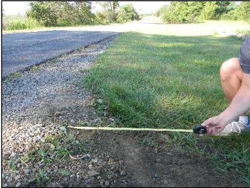
The mailbox post should be positioned so the front of the mailbox will be set back 6-8" from the face of the curb (or the edge of the road) to the mailbox door. To determine the location of the Ground Post, mark the desired set back position to the front of the mailbox and add 28-inches. This should place the Ground Post off the roadbed surface by about 34 to 36-inches. Further set back can be provided if the carrier can safely pull off and re-enter the roadway.
