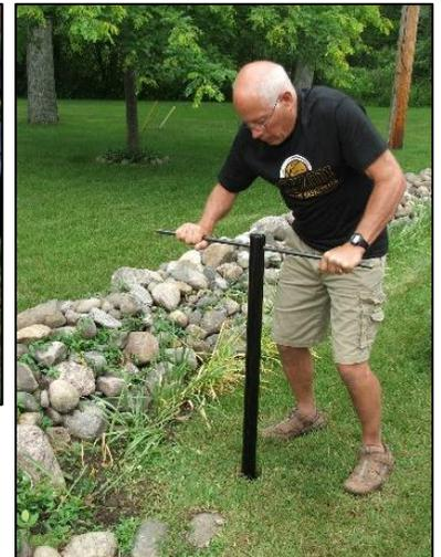
**Note:** *If the ground is very dry or hard and obtaining auger penetration is difficult, you may try to pour water directly down the Ground Post and/or around the post base. This usually works well.*
