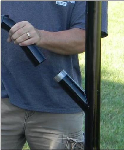
5. Place the assembled Mailbox Mounting Arm (Part 5) onto the Receiver Post of the Rotating Self-Centering Pipe. Check the vertical alignment of the Mounting Arm with that of the Ground Post. When satisfied with the correct orientation, tighten the u-bolt nuts on the Mounting Arm securely and then firmly set the Mailbox Mounting Arm onto the Receiver Post of the Rotating Self-Centering Pipe Assembly using a rubber mallet or hammer and board. Firmly tighten the bolts on the Mounting Brackets.
